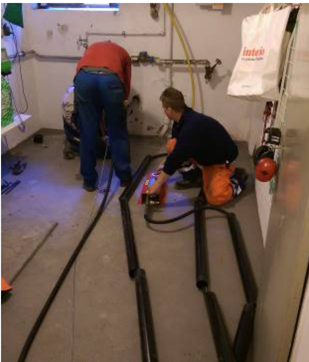
The Hauff-Zappo pipes 1 m long (3.3 ft) are easily connected together.
