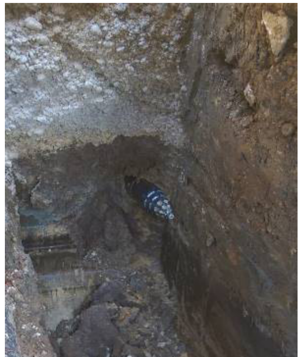
The TERRA-HAMMER T 080mini SK arrives at the target pit very precisely.
