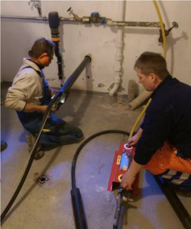
The TERRA-HAMMER T 080mini SK with end sleeve Ø 90 mm is installed in the cellar.
