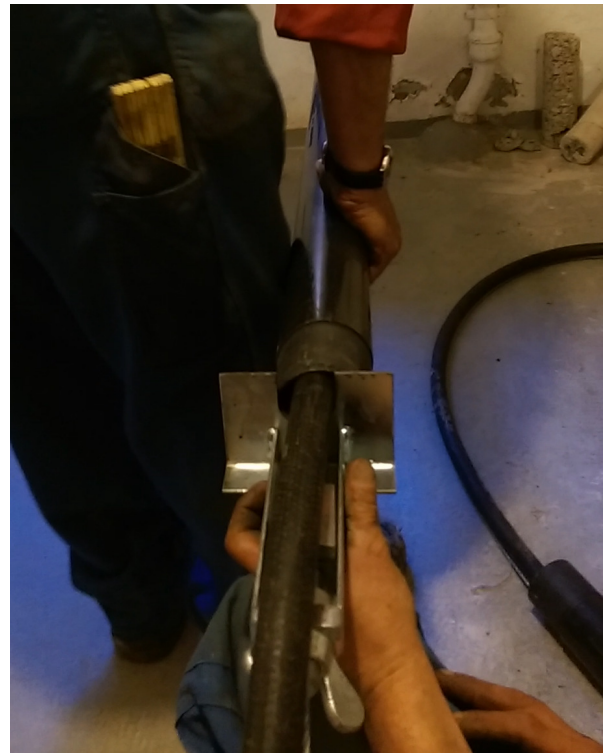
The pipe Ø 75 mm from Hauff-Zappo is fixed with the cable clamp.
