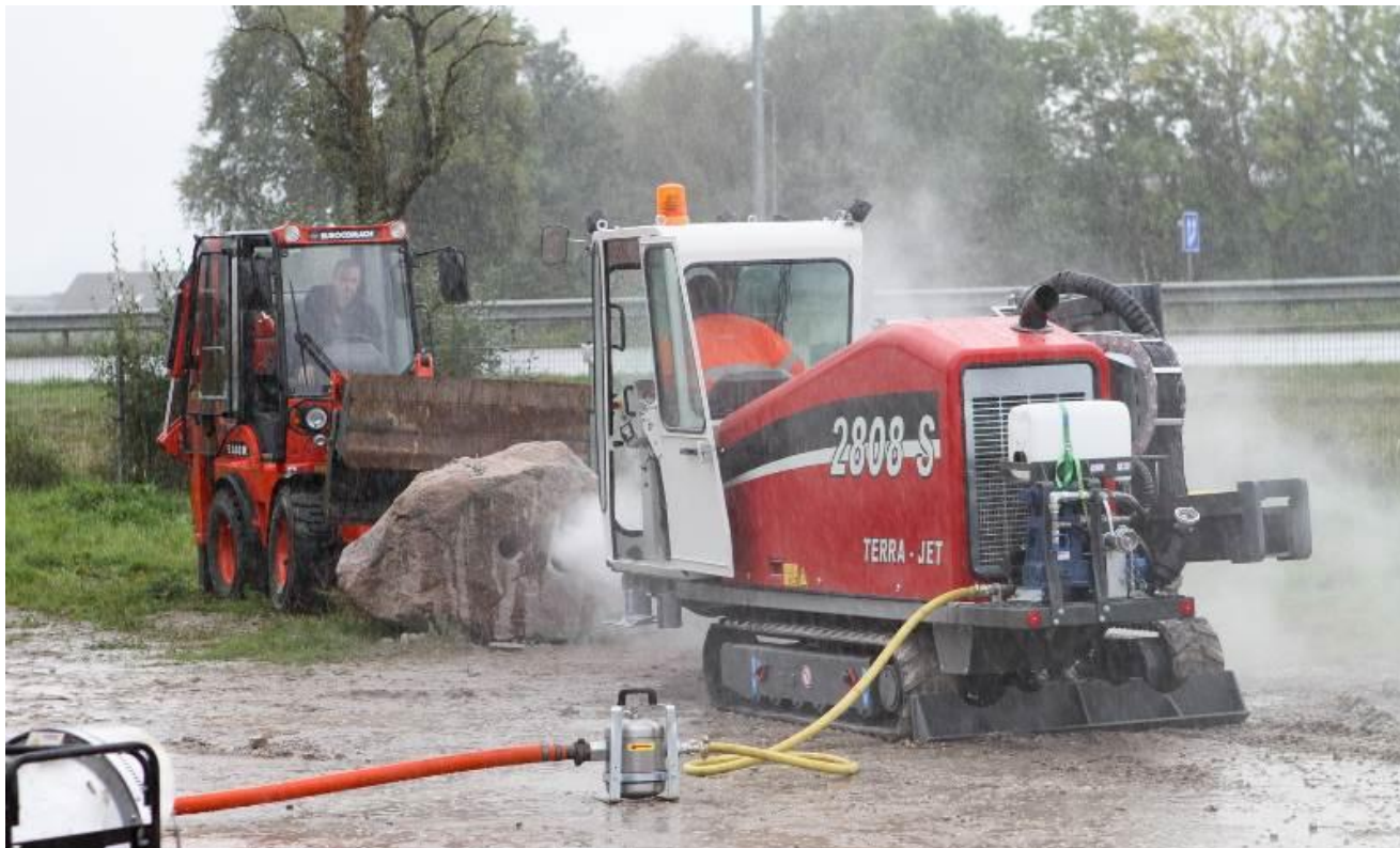
Pic. 7: It took only 13 min to drill through the granit bolder
