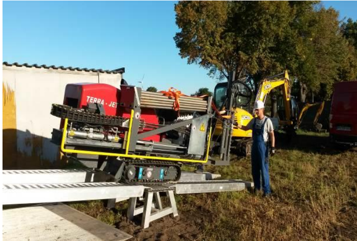
Pic 1: The 4 tonnes HDD machine is moving out of the truck.
