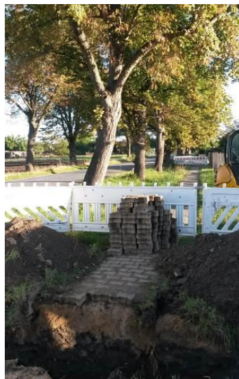
Pic. 3+4+5: The ground was filled with stones, concrete and other obstacles down to a depth of 2 m (6.6 ft). Deeper they found sandy clay.
