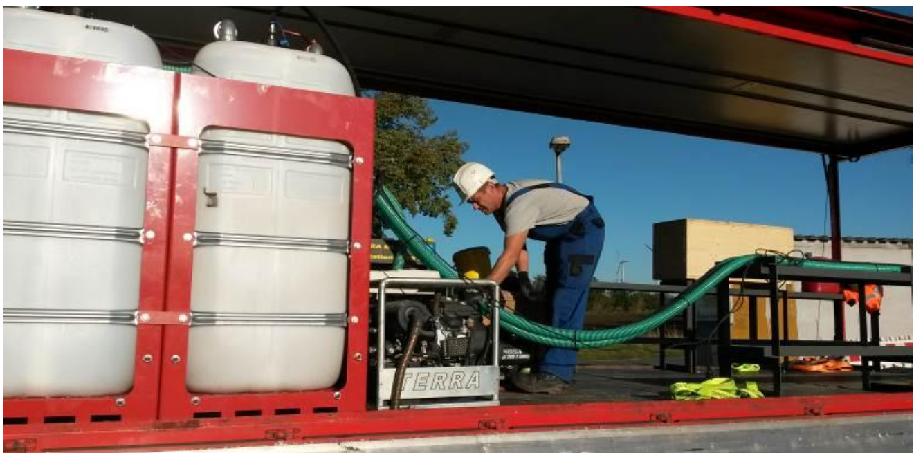
Pic.2: The complete mixing and pumping system is on the truck.
