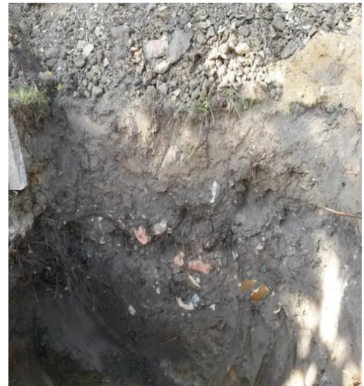
Pic. 3+4+5: The ground was filled with stones, concrete and other obstacles down to a depth of 2 m (6.6 ft). Deeper they found sandy clay.
