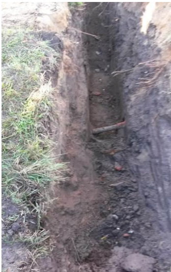
Pic. 3+4+5: The ground was filled with stones, concrete and other obstacles down to a depth of 2 m (6.6 ft). Deeper they found sandy clay.
