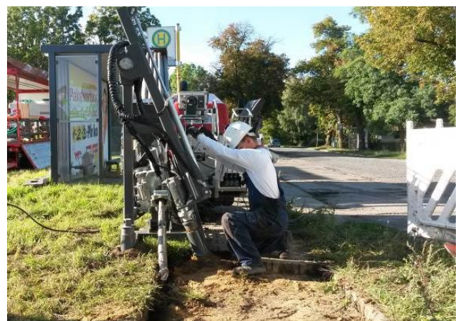
Bild 6+7: The TERRA-JET in drilling position. Due to the extreme entry angle of up to 67% the required drill depth could be reached immediately. The anchoring with the two ground anchors is fast and easy.
