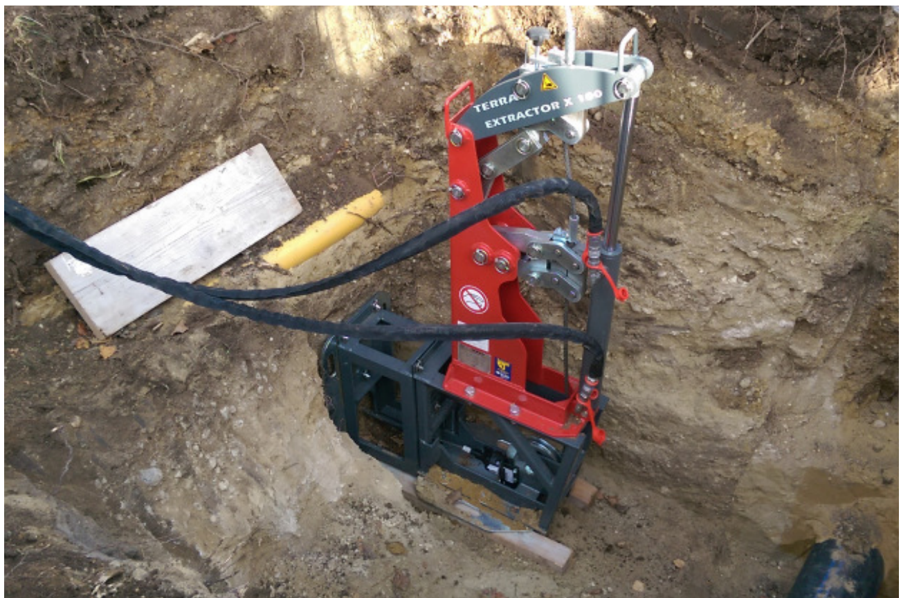
Pic. 3: At the machine side the cable is assembled through the pipe burster. The bursting length was 12 m (40 ft). It undercrossed the pathway and the front garden of the house.
