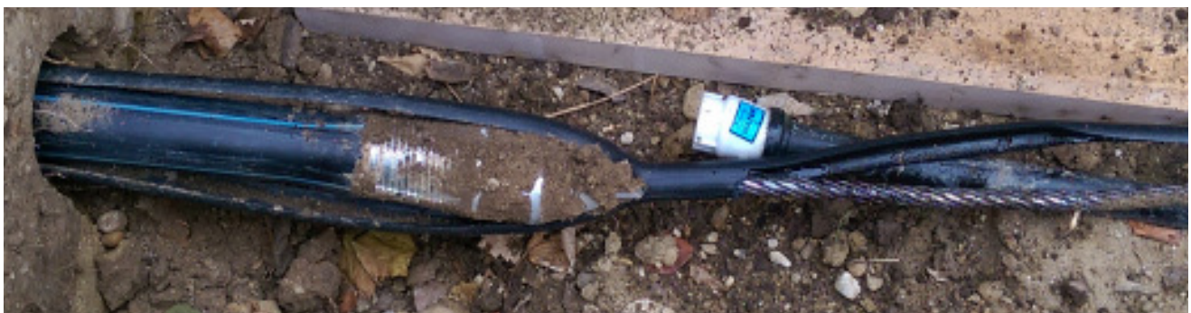
Pic. 5: View on to the new HDPE pipe OD 40 mm (1.5") and the old cut PE pipe after the disassembly of the TERRA-EXTRACTOR X 100. The renewal of the house connections in Weiden were finished without interruptions, the contractor Altenthaler Bau GmbH could realize several new house connections per day including the connection to the main water line, which was continuously under pressure. So the house owners were cut off from fresh water only for half a day.
