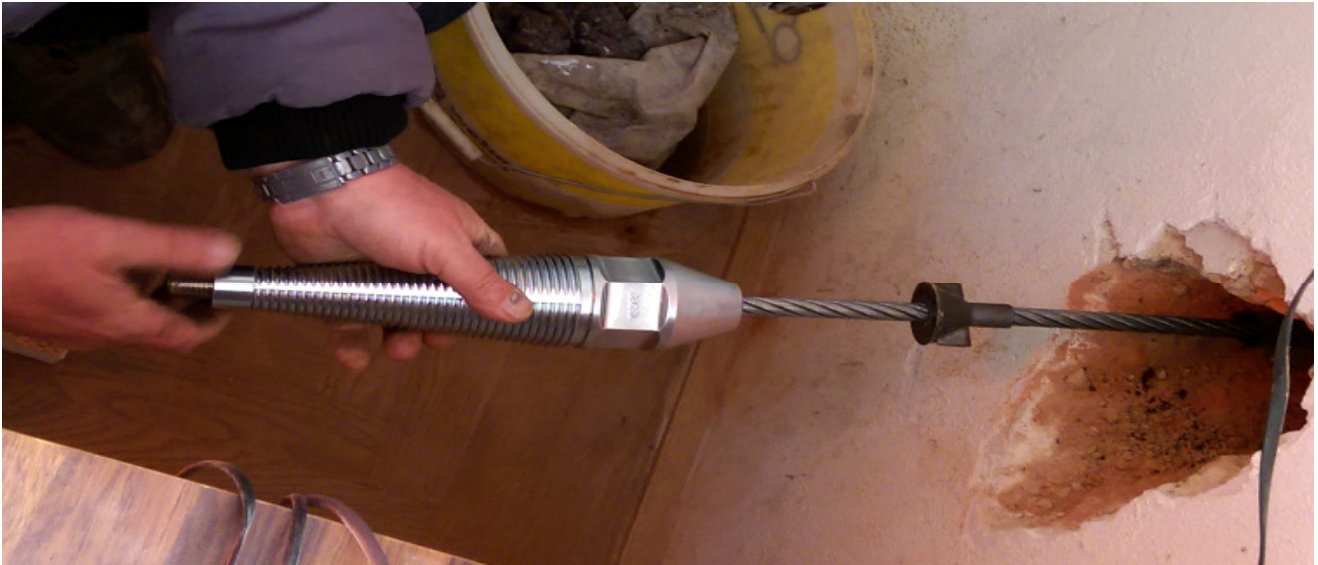
Pic. 2: In the cellar the old pipe is cut off from the installations inside of the house. The wall around the old pipe is opened. Then the PE cutter and the connector for the new HDPE pipe are assembled.
