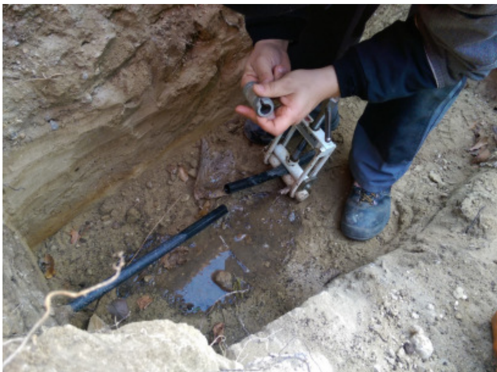
Pic. 1: The compact Cable Burster requires a minimum space of 0.65 x 0.40 m.
