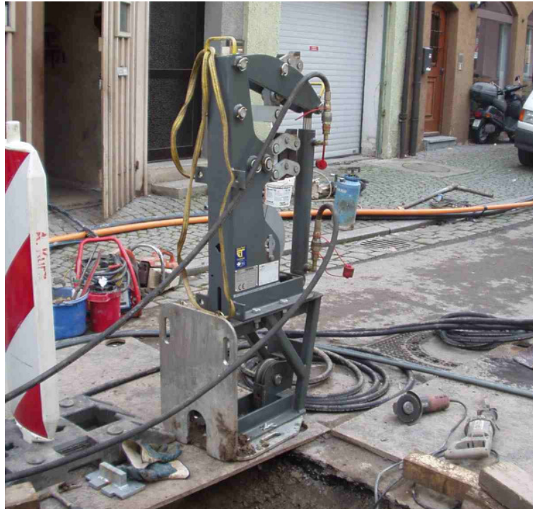
The TERRA-EXTRACTOR X 100 is prepared to be lifted into the pit.
