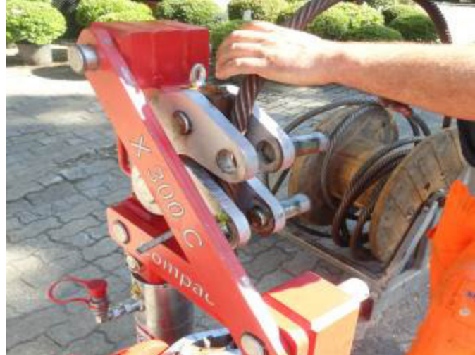
The pulling cable is inserted into the cable burster.
