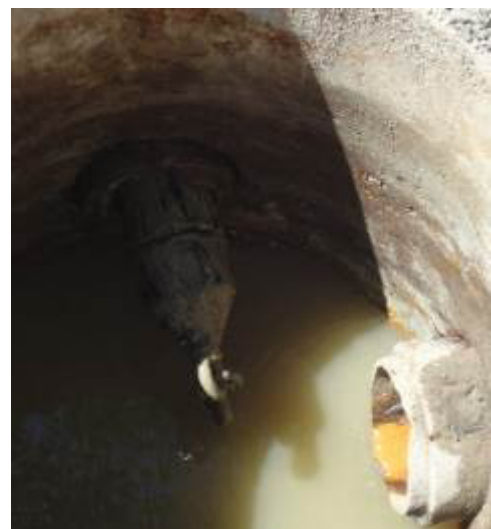
← The new HDPE pipe OD 125 mm (5") is pulled in.
