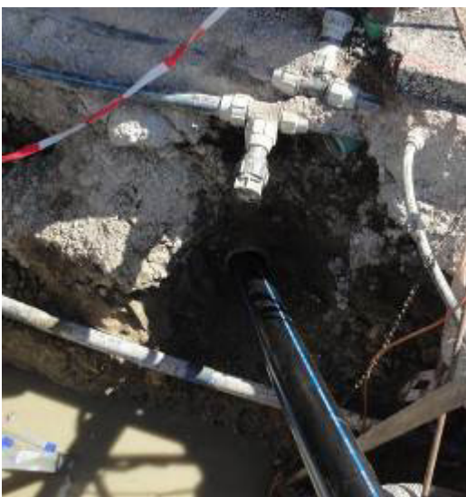
← The new HDPE pipe OD 125 mm (5") is pulled in.
