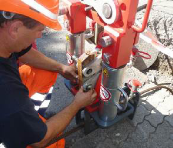
The pulling cable is inserted into the cable burster.
