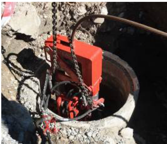
The TERRA-EXTRACTOR X 300 C in the manhole Ø 1.0 m (3.3 ft).
