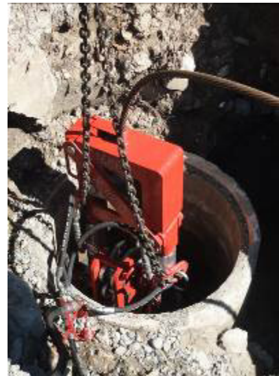
→ The X 300 C during pipe pulling. The speed was between 25-30 m/h (80-100 ft/h).
