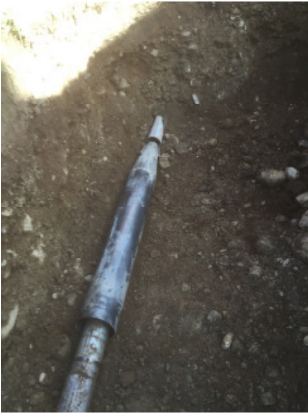
Picture 2: The TERRA-HAMMER T 105 S is slid into the expander Ø 170 mm (6.7").
