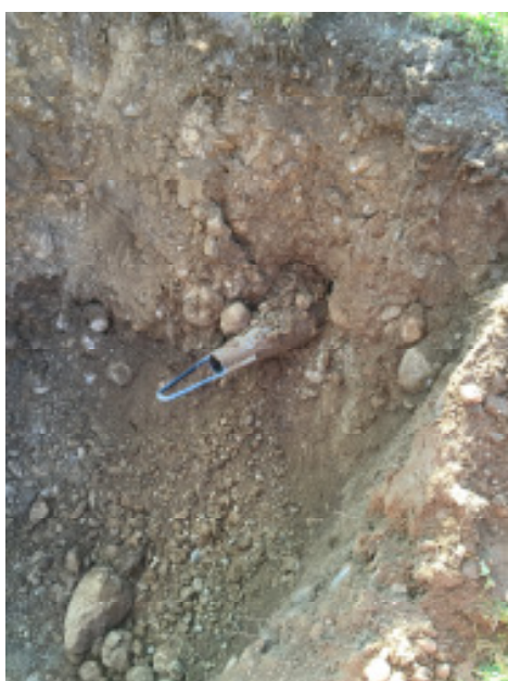
Picture 5: The expander reaches the arrival pit.
