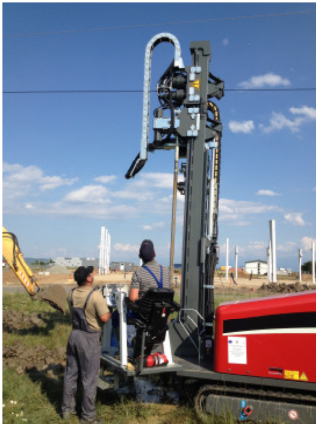
Picture 6: The TERRA-JET TJ 2808 S during vertical drilling.
