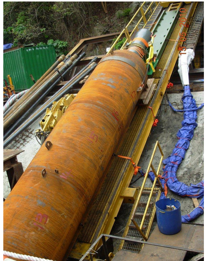
The TERRA-HAMMER TR 565 during the ramming.
